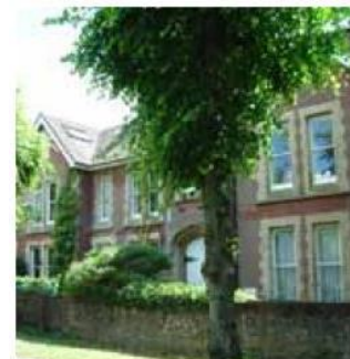
Older property converted to five dwellings
