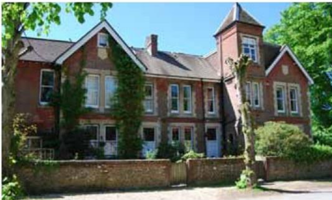
Older 3 storey property converted into five dwellings
